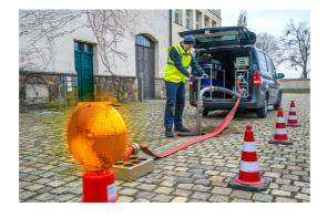
Flushing drinking water networks efficiently with conditionbased network flushing In recent years, TZW has developed the methodology of condition-based network flushing as a result of research and consultancy projects. Positive practical experience has led to this approach being taken into account in the revision of DVGW rule W 291. Condition-based flushing is already being implemented in practice at German water supply companies in Chemnitz, Leipzig and at RWW.
